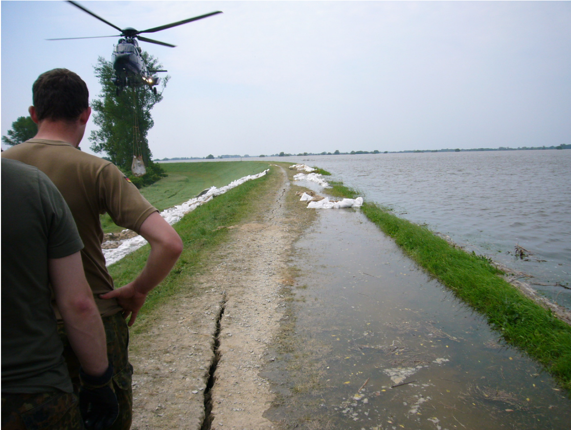
Figure 1: Dike at the river Elbe close to Fischbeck on June, 9 – 10 hours before the break (Ellmann, 2013)
