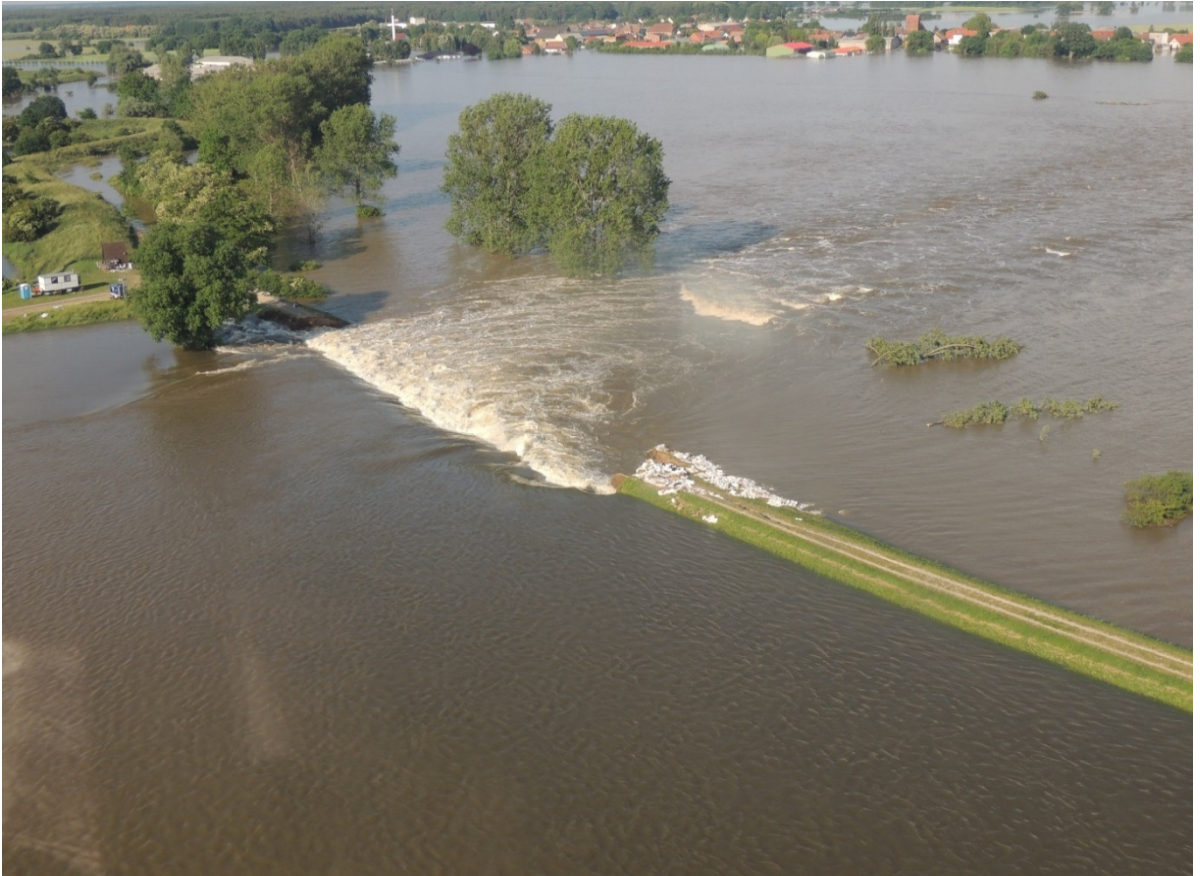
Figure 2: Dike break at the river Elbe close to Fischbeck on June, 10 – 18 hours after the event (Juepner, 2013)
