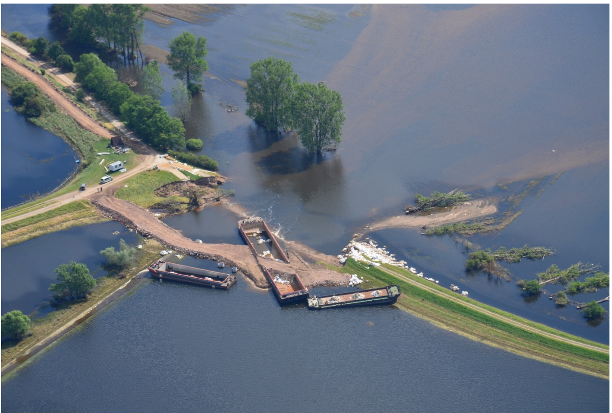
Figure 3: Dike break at the river Elbe close to Fischbeck on June, 22 – 12 days after the event (Mueller, 2013)
