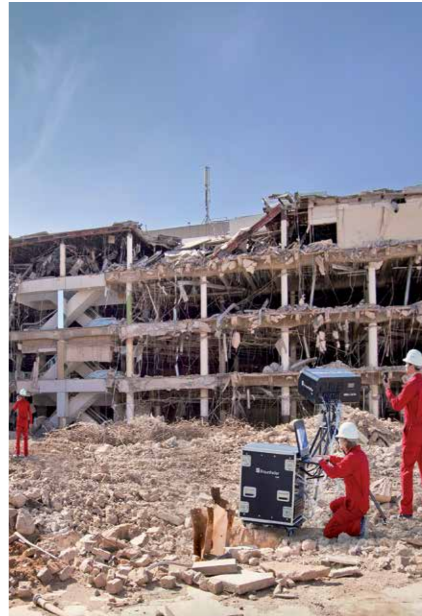
Collapsed structures after earthquake: Typical scenario for application of RAWIS warning system. © Fraunhofer FHR / Uwe Bellhäuser
