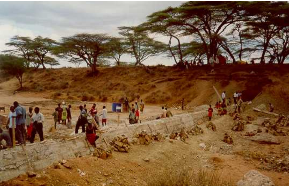
Figure 5 Building sandbanks on Baragoi River, Samburu
