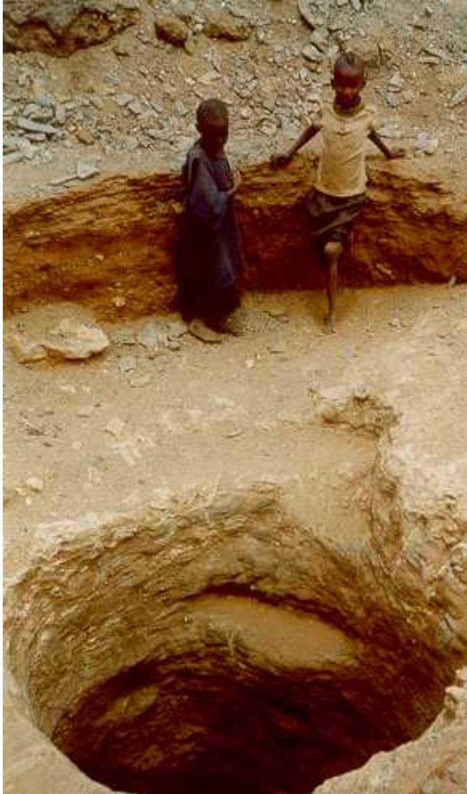
Figure 3 Hand dug well in Baragoi River, Samburu
